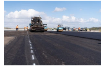
Equipment being used to add the final layer of runway pavement
