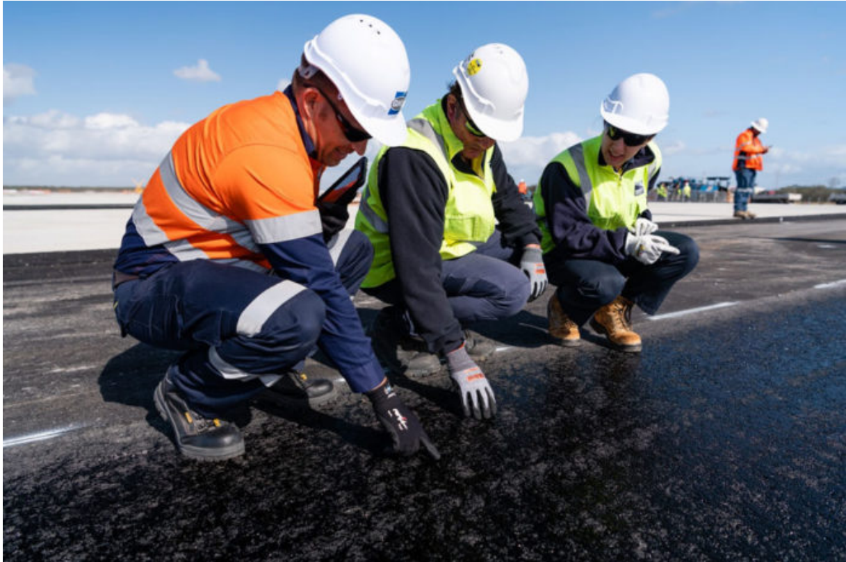
Workers inspecting the new layer of runway pavement
