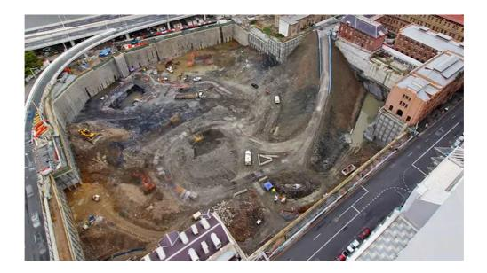
▲ Queen's Wharf Development: The giant hole in the ground, down to a depth of 26 metres at its deepest will be transformed into Queensland's largest basement and underground carpark.
