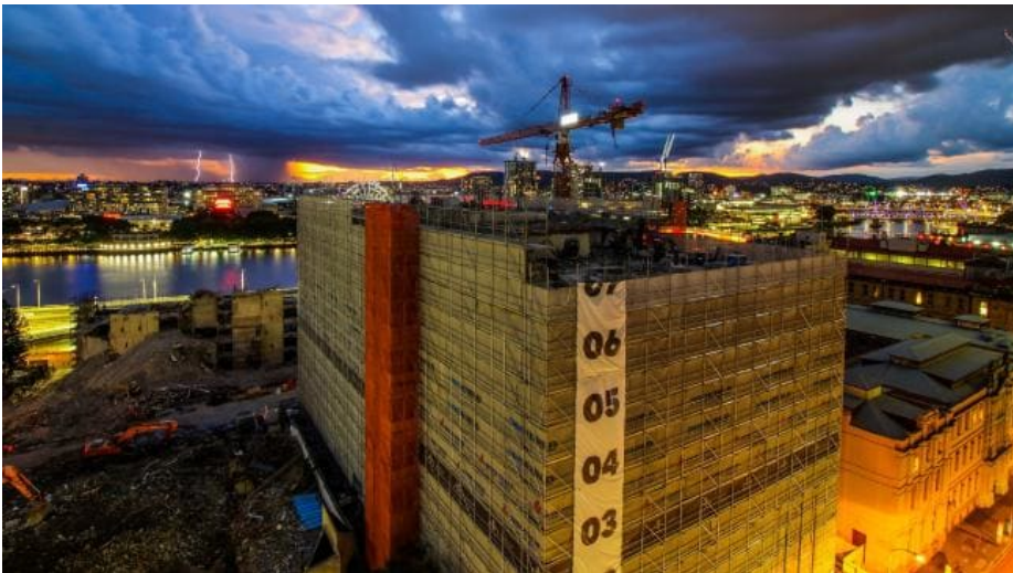
The Queens Wharf development under construction in Brisbane’s CBD. Source:Supplied
