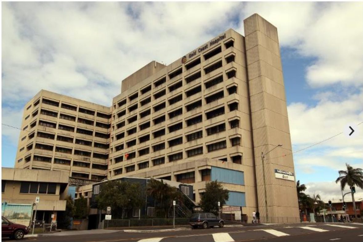
📷 The former Gold Coast Hospital at Southport before demolition began.
